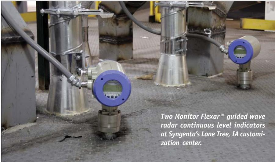
*Two Monitor Flexar™ guided wave radar continuous level indicators at Syngenta's Lone Tree, IA customization center.*
